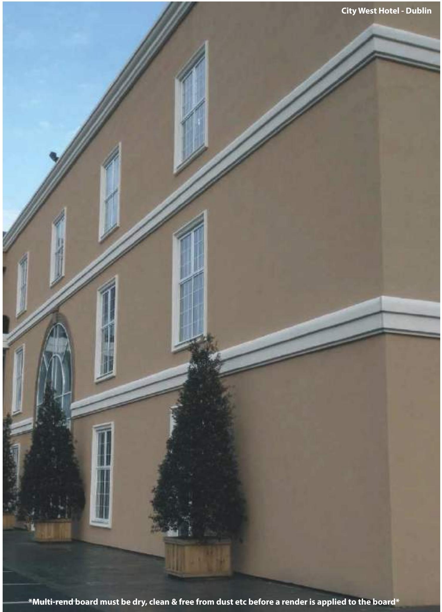
**\*Multi-rend board must be dry, clean & free from dust etc before a render is applied to the board\***
