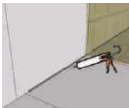
6. Run a bead of silicone along the internal joints before tiling and then again after the tiles are fitted - this is standard fitting procedure. (Tanking recommended when tiling wet rooms.)
