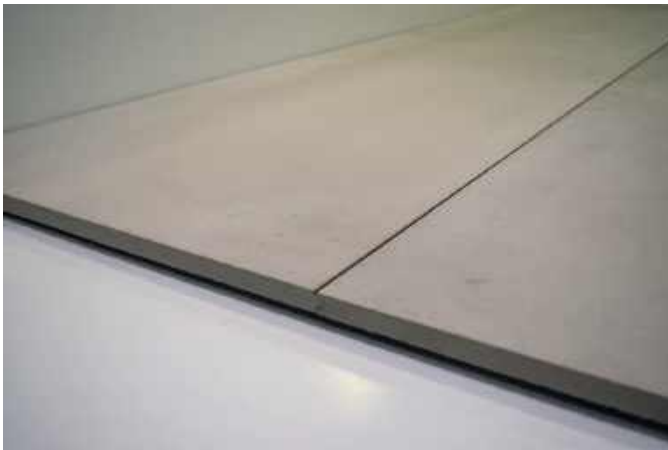
Figure 1: flooring boards fitted logo face down and T & G expansion profile gap up
