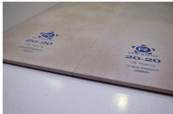
Figure 2: flooring boards logo fitted face up with T & G expansion profile gap down
